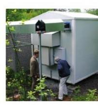
thermal insulation. The cabinets are light, strong and weatherproof, but indoor mounting offers the best protection against weather and vandalism. The units use through-wall air intake and can be wall, floor or roof-top mounted.
